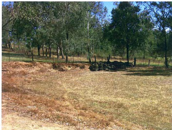
Photograph 13: Cut area and tyre stockpile in Lot 44.
