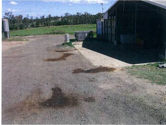
Photograph 16: A 200 L drum located on a concrete block outside a storage shed on Lot 3 in DP230943. Oil staining on the gravel driveway between the storage shed and chicken sheds.
