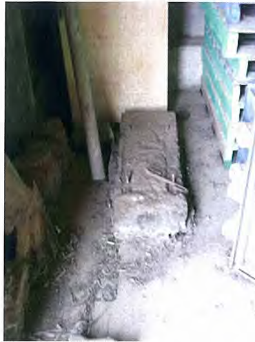
Photograph 5: Concrete pad with protruding bolts.
