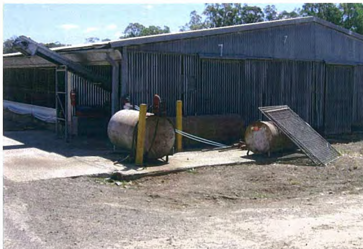
Photograph 7: ASTs located adjacent to shed 4. Diesel staining is visible on the underlying concrete slab.
